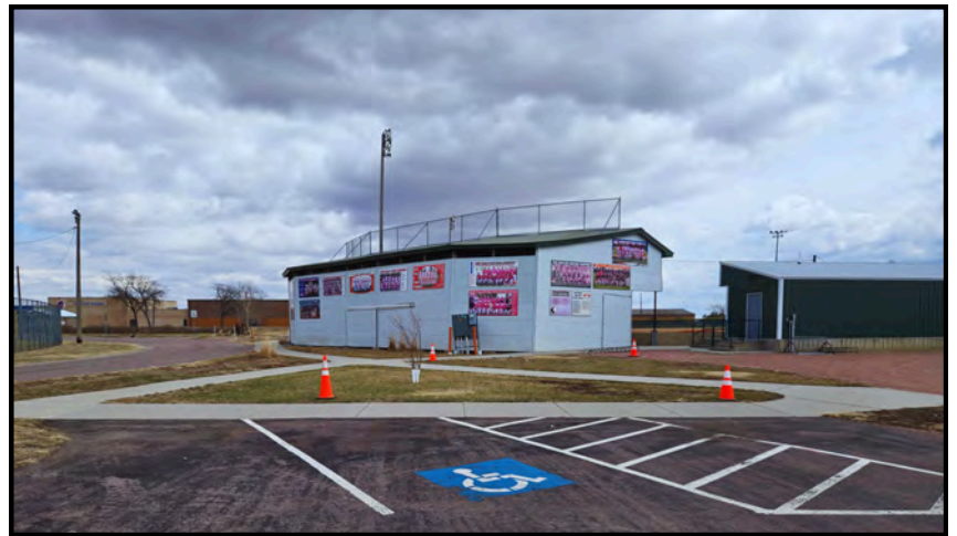
Future building site Looking East from the nearby small parking lot "The Pond" shown in the background
